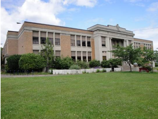
East elevation entry
