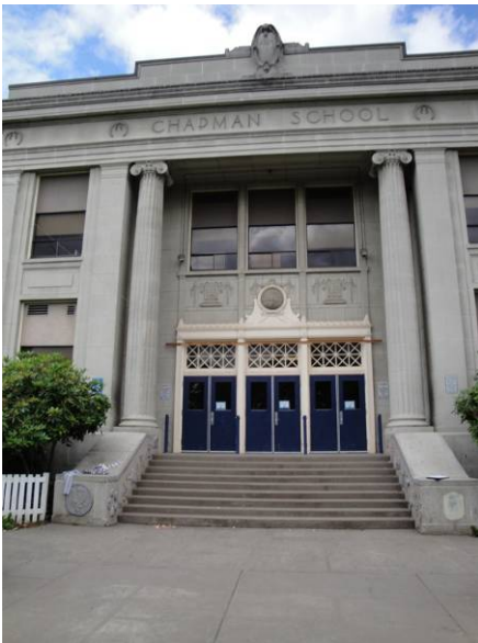
East elevation entry
