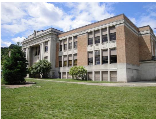
East elevation entry
